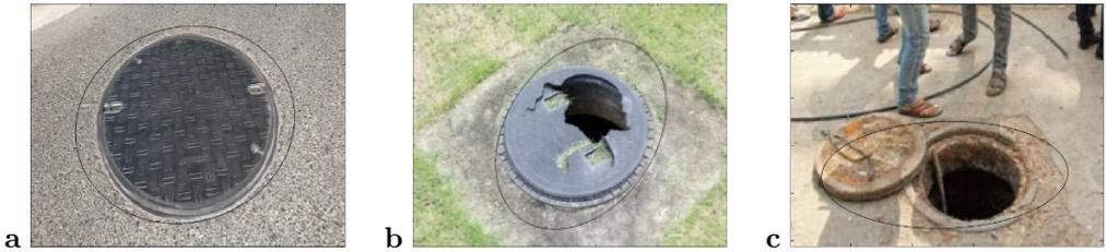
Fig. 5. Samples of the ellipse drawn by the algorithm around each class: (a) closed, (b) broken, and (c) open manhole.
